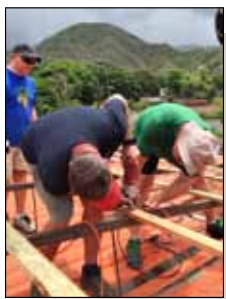
Adults install a church roof in Jamaica.
